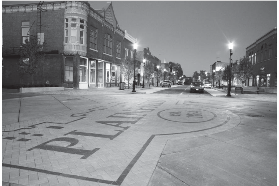
Plainfield's Lockport Street Complex, an award-winning project worked on by The George Sollitt Construction Company. Below at right, another award-winner, Clark Construction Group's 300 N. LaSalle.
